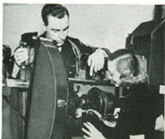
Mechanical scanning camera used by Dr. E. F. Alexanderson about 1930.
