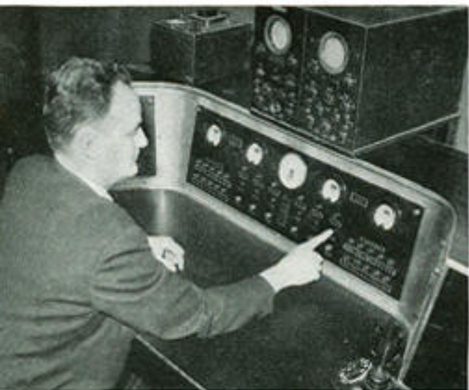
Master control board of NBC's television transmitter station, located on the 85th floor of the Empire State Building.
