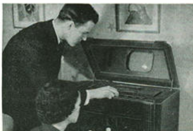
Close-up of receiver; Kinescope image is reflected onto mirror under lid.
