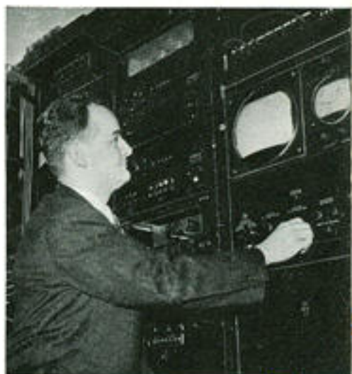
Section of transmitter control board in the Empire State Building.
